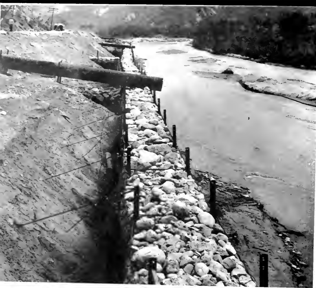
Steel rail and cable and rock-fill double fence bank protection
